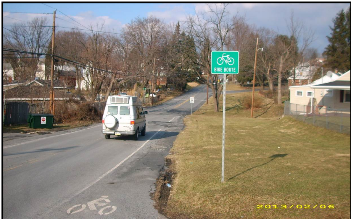
Photo 9: Parkway Drive looking north within the City near Walnut Street.
