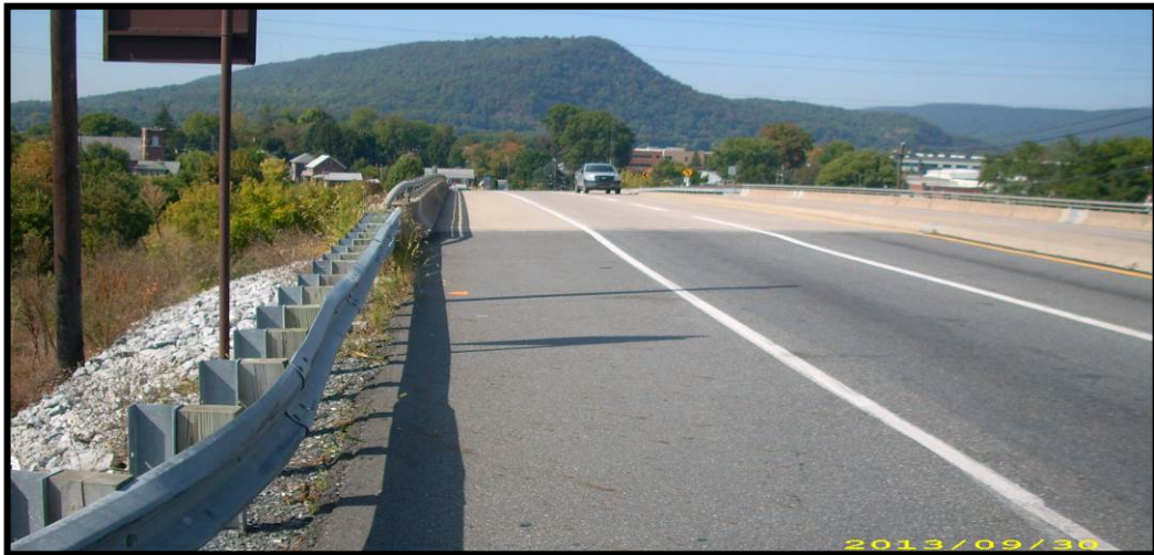
Photo 17: South side of bridge, shoulder for trail location in Option B.
