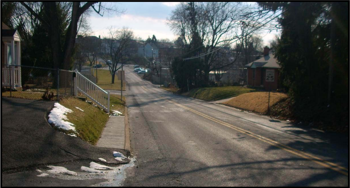
Photo 10: Parkway Drive looking south from the Township near Herr Street.
