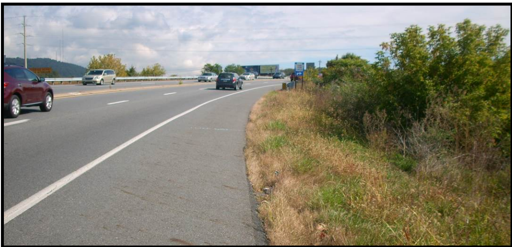
Photo 18: Linglestown Road shoulder approaching the bridge from the west.
