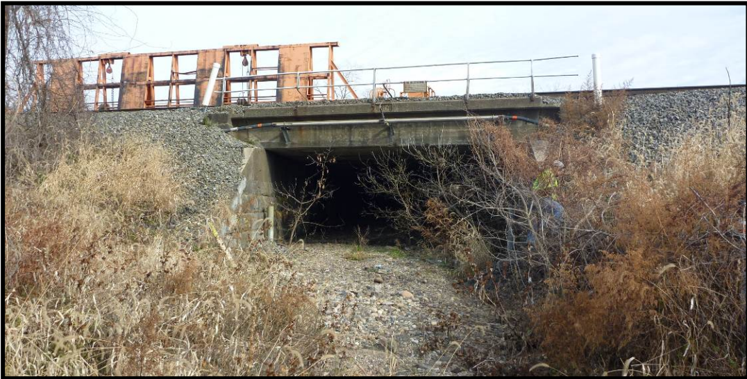
Photo 13: West face of the railroad underpass (old Linglestown Road) – Option A.
