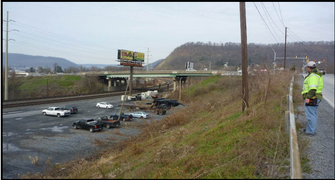
Photo 11: Industrial Road looking north towards the Linglestown Road bridge over the railroad. This is a view of the Option A alignment.
